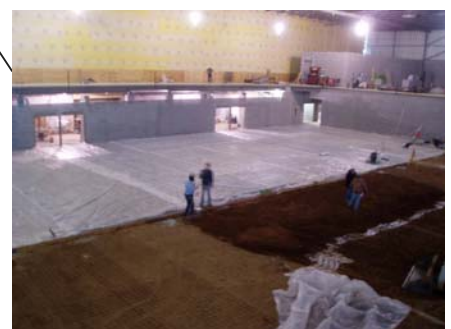
Half of the Gym Slab has Concrete Poured
